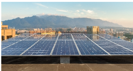
Commercial building & factory rooftop
