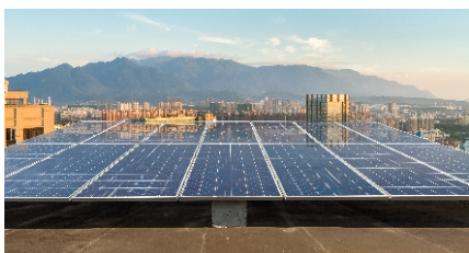
Commercial building & factory rooftop
