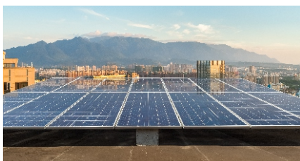
Commercial building & factory rooftop
